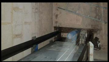
After removing and disposing of the old lift equipment, the survey our lift expert completed found insufficient fixing points to handle the lift load. Due to part of the brief including the lift shaft being hand painted with bespoke black metallic paint, and LED mood lighting to enhance the metallic effect.
