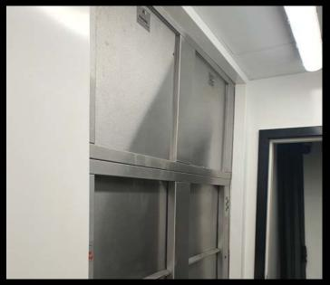
In our building accessibility specifications, our VT engineers specified products that used leading industry components to provide open protocol systems for the lifts. Which were, two MRL, 1000kg, 13 person lifts utilizing iKONIC Mars Passenger Lifts. IKONICs Goods-Only Passenger Lift for basement goods storage.
