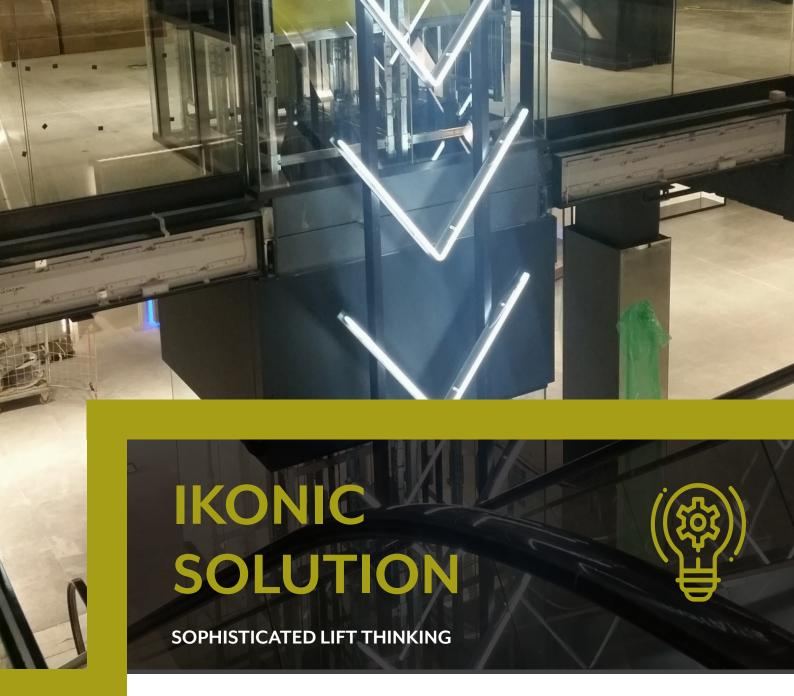
The product iKONIC chose was particularly appealing to the client due to it being 8 person and travelling at 1 m/s. the lift was finished with framed glass fire rated doors and a counterweight safety gear due to the suspended pit.
